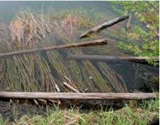
PHOTO 1: SOAKING CUTTING AT OR NEARBY INSTALLATION SITE
