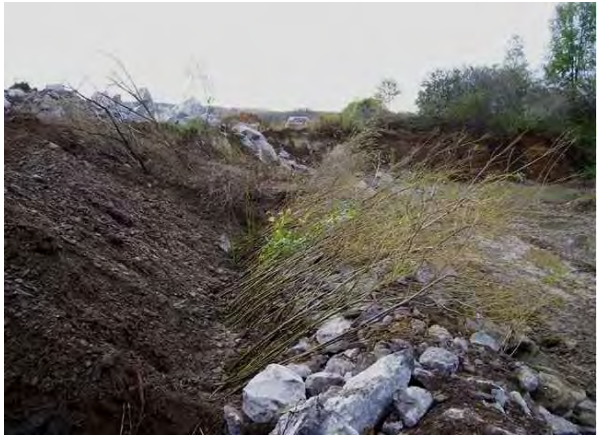
PHOTO 2: BRUSH LAYER PRIOR TO BACKFILLING AT TOE OF SLOPE (OTHER ASPECTS OF THIS EXAMPLE DIFFER FROM THE DETAIL, E.G. ROCK BASE INSTEAD OF COIR LOG)
