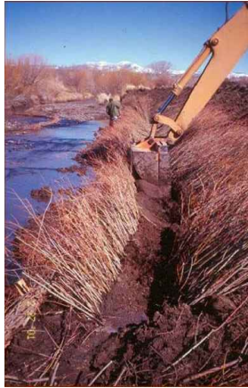
PHOTO 4: EXAMPLE OF LIVE SILTATION BRUSHLAYER BEING BACKFILLED, WITH ADDITION OF VERTICAL BRUSHLAYER ON LANDWARD SIDE OF TRENCH
