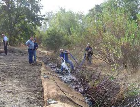
PHOTO 3: WATERING IN AS BACKFILLING OCCURS (OTHER ASPECTS OF THIS EXAMPLE DIFFER FROM THE DETAIL, E.G. ANGLE OF BRUSH LAYER AND USE OF COIR CLOTH)
