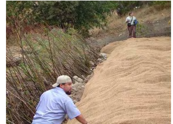
PHOTO 5: EXAMPLE OF BACKFILLED TRENCH IN SLIGHTLY DIFFERENT SETTING (OTHER ASPECTS OF THIS EXAMPLE DIFFER FROM THE DETAIL, E.G. NO COIR LOG AND USE OF COIR CLOTH)
